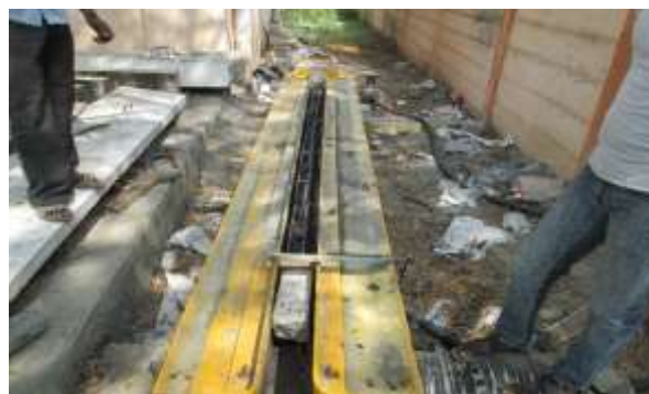
Fig.1 Steel reinforcement placed in the mould
